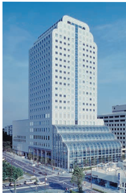
Outside of Senri Life Science Center Building at completion of construction
